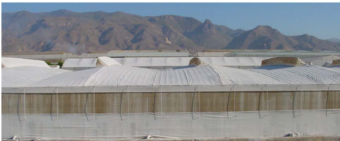
Figure 6. Side-wall and zeneral openings, all netted, in a parral greenhouse in Almeria, ES. The permeability of the nets may be further reduced by accumulation of dust.
