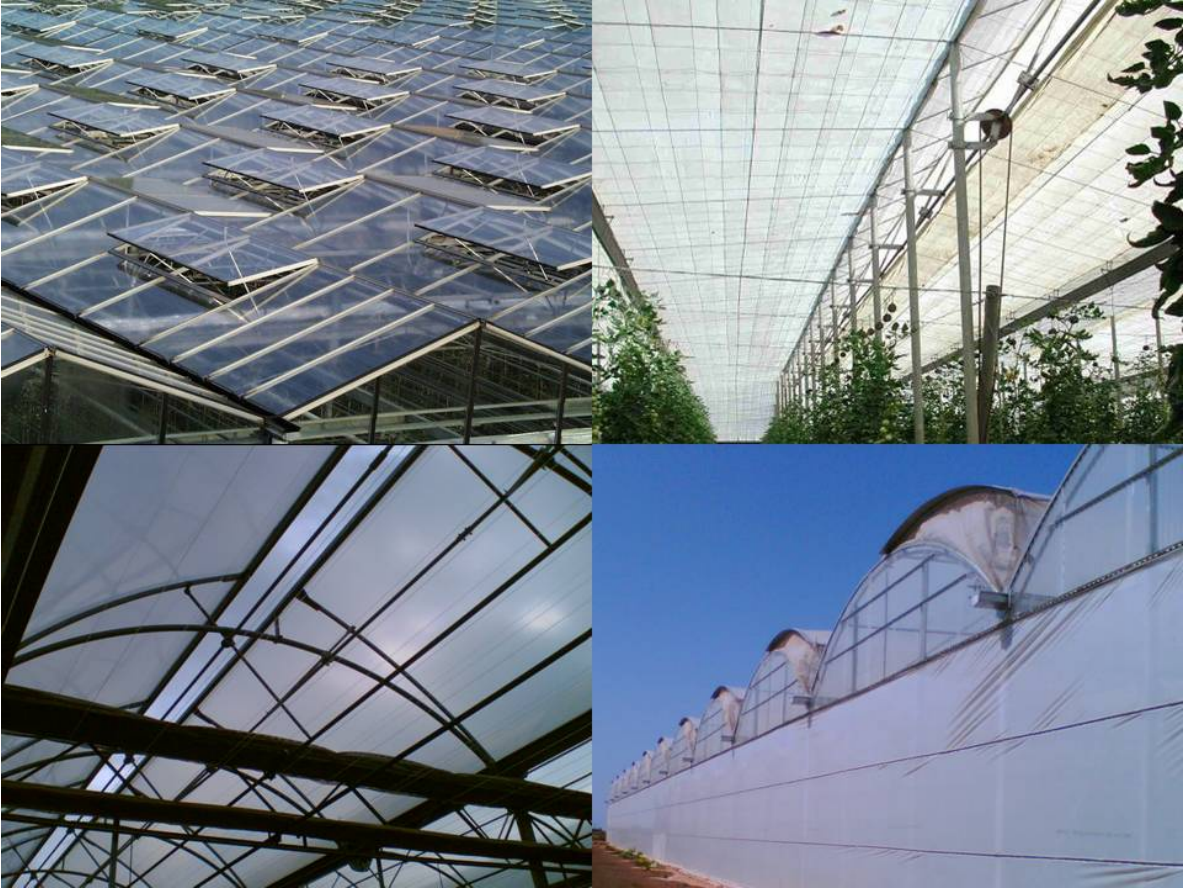
Figure 4. Examples of regulated ventilation openings in greenhouses. Clockwise from top left: alternate ridge openings in a Venlo glasshouse, Holland; parallel greenhouse with one-side ridge flap, Almeria, ES; multitunnel with 'seagull wing' openings, protected by insect nets, Sicily, Italy and fully retractable roof, Barcelona, ES.
